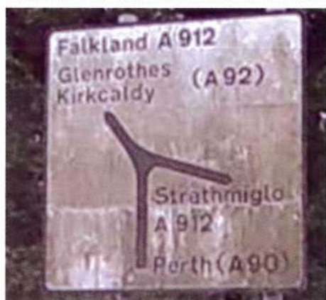
Before -洗浄後に施工-
